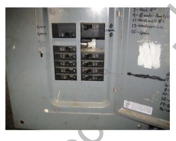
Has 2 double lugged breakers, add 2 breakers & separate the (2 wires) double lugged breakers to 1 wire per breaker.
