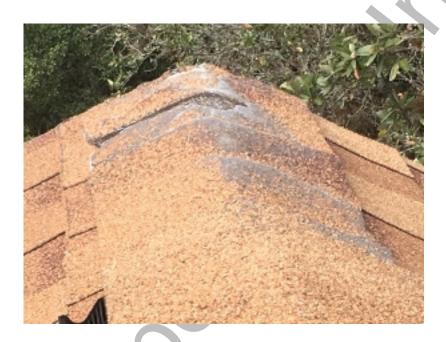
■ THERE ARE MULTIPLE DAMAGED / WORN RIDGE CAP SHINGLES – At various locations.
