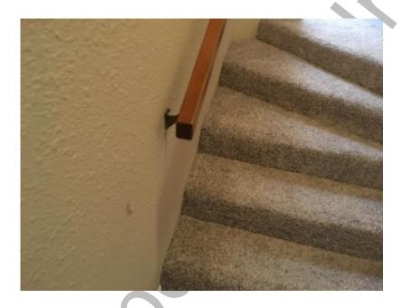
■ A PROPER HANDRAIL IS NOT PRESENT — At the rear porch & the bottom flight of stairs. The handrail grip size shall be a minimum of 1 ¼ inches to a maximum of 2 5/8 inches.
