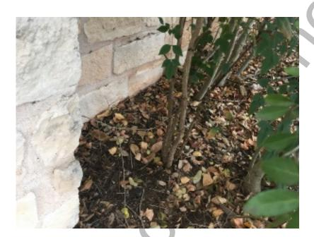
Regrade the soil down & away from the foundation (the code requires 5% slope extending 10 ft. out from the house) to divert the water around & away from the house, especially at the right rear. In other words, this means that the soil should fall 6 in. within 10 ft. of the house on all 4 sides of the house.
