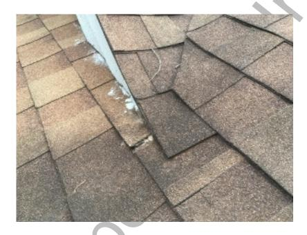
■ THERE IS AN EXPOSED ROOF NAIL – Through the surface of the shingles at the rear of the valley above the garage.
