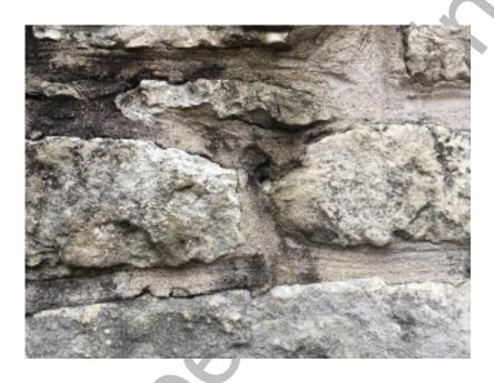
■ WEEP HOLES EVERY 33 IN. – Are missing at the first layer of the rock & above the door & windows at various locations.
