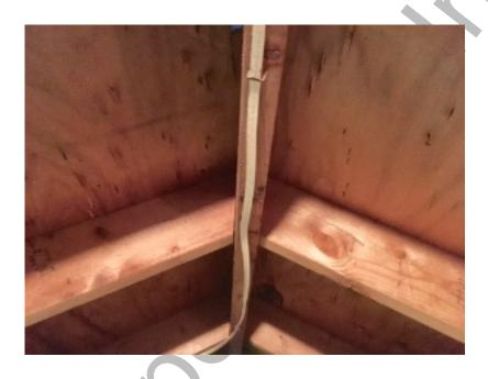
■ THE ATTIC DOOR (PULL DOWN STAIRS) – Cut the legs of the stairs so that the stairs are straight & the hinges are properly engaged. The garage attic door is not a fire rated door.
