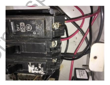
ARC PROTECTION BREAKERS FOR ALL LIVING AREAS (AFCI – ARC FAULT CIRCUIT INTERRUPTOR BREAKERS, WHICH ARE FIRE PREVENTION DEVICES) – Are now available (required as of the 2009 code).  $\boxtimes$
