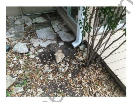
■ REGRADE THE SOIL – To expose 4 to 6 in. of the slab at the right rear & the left front of the living room.
