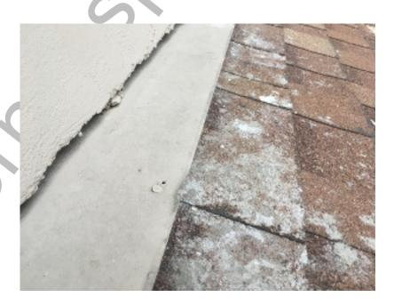
ALL EXPOSED ROOF NAILS - Are not sealed (caulked) at the flashings, roof vents & ridge shingles to prevent water penetration.
