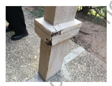
■ THE POSTS / PIERS FOR THE OBSERVATION DECK — Have concrete poured around them, which can trap water against the posts / have wood to ground contact. The concrete is cracked / damaged.
