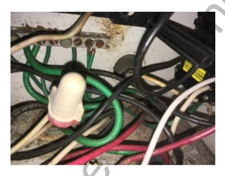
■ The box has 2 double lugged breakers, add 2 breakers & separate the 2 wires on the double lugged breakers to 1 wire per breaker.
