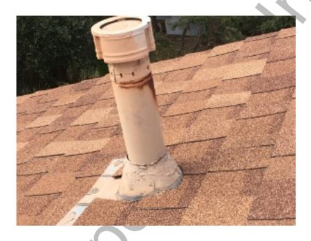
■ THERE ARE LOOSE / RUSTED FLASHINGS – At various locations including at the skylight, the left rear & the chimney.
