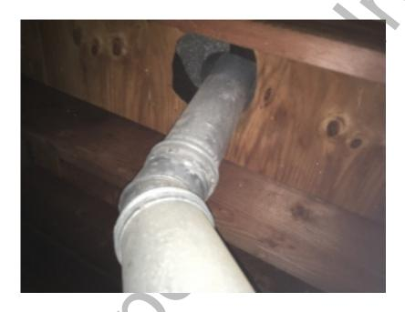
■ THE VENT PIPE RAIN COLLAR – Lower the rain collar down to the flashing cone & reseal the rain collar to the vent pipe to prevent water leakage into the attic above the garage.
